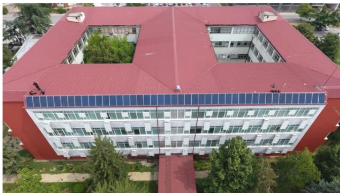
Fig. 4. INNOFEIT Living Lab 30 kW solar power plant
