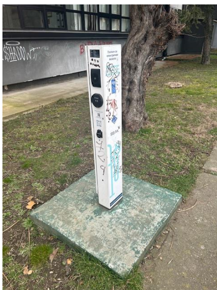
Fig. 6. INNOFEIT Living Lab 24 kW electrical vehicle charger
