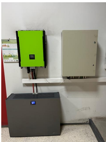
Fig. 5. INNOFEIT Living Lab inverter and battery storage
